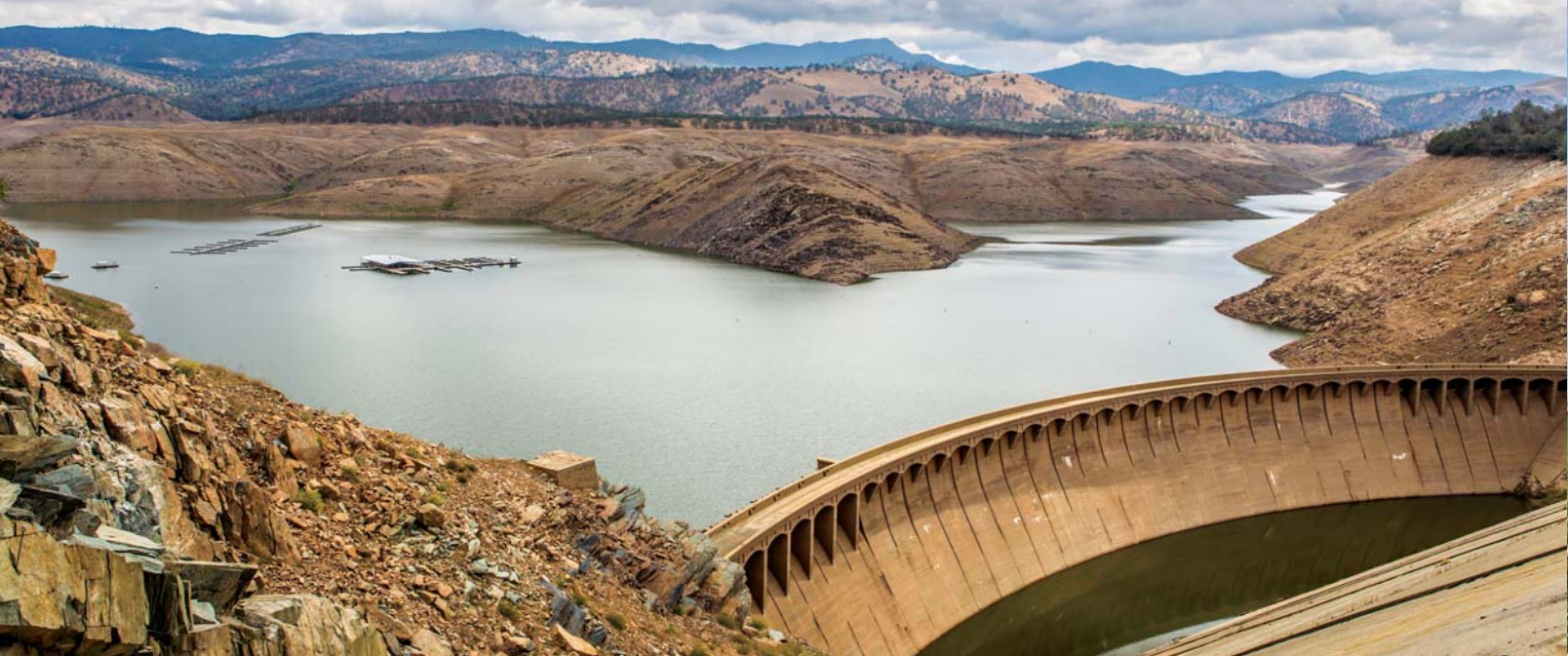
California's Lake McClure, just northeast of Fresno, dropped to 10% of capacity in 2015. The drought revealed huge cracks in the ground where there should be 200 feet of water depth.
